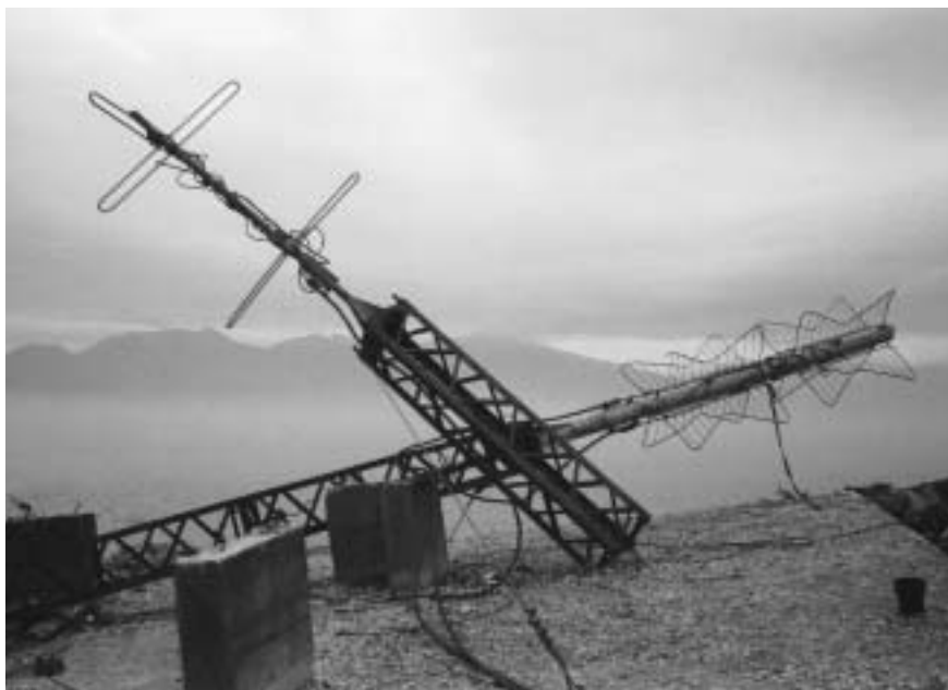
A radio and TV transmitter lie scrapped on the hills above Kabul after the U.S. bombing in fall 2001 destroyed transmission facilities.
